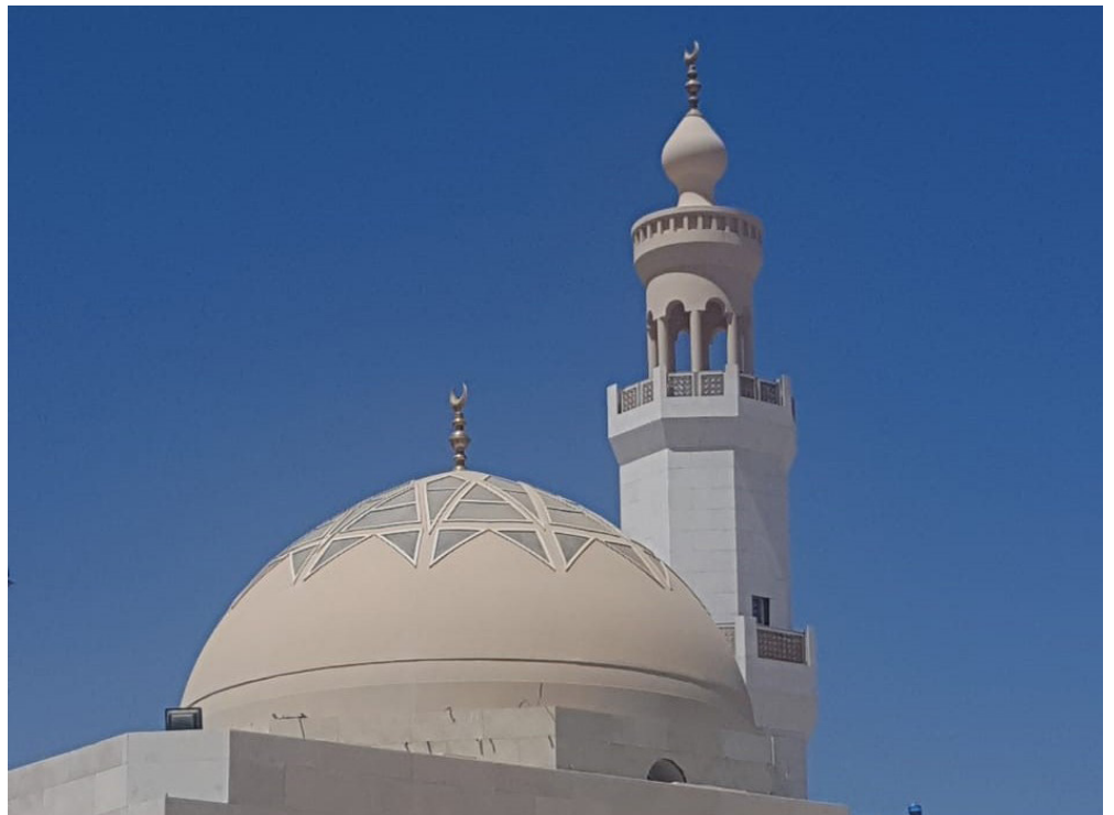
Final shot of the minerate after completion.
