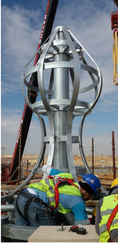
Galvanized Steel Frame for the top part of the minaret.
