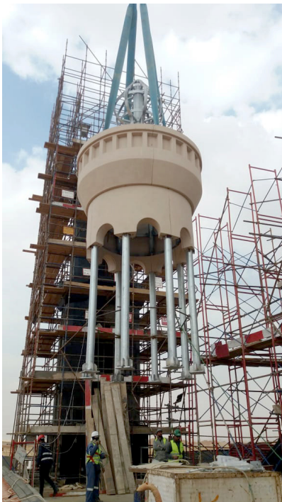
Lifting the minaret's balcony to its position from the ground.
